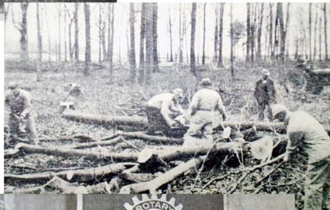
Building the 4-H Park
